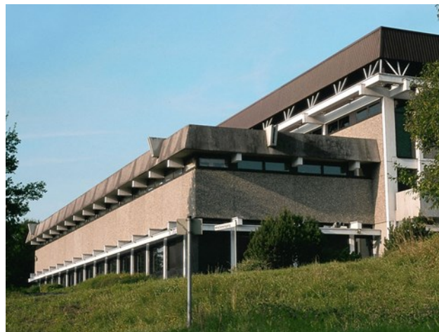
Neckarhalle Am Park 10, Obrigheim
